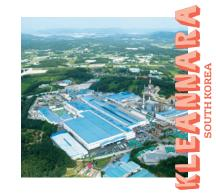
The Korean paper manufacturer KleanNara has entrusted Veolia with the management of water treatment (59,000 m<sup>3</sup> of water per day) and wastewater (28,000 m<sup>3</sup> per day) facilities on its Cheongju site. The Group also operates two boilers, producing 42.5 metric tons of steam per hour; the solid fuel used comes from the plant's production process. This circular economy loop significantly reduces the plant's environmental footprint.
