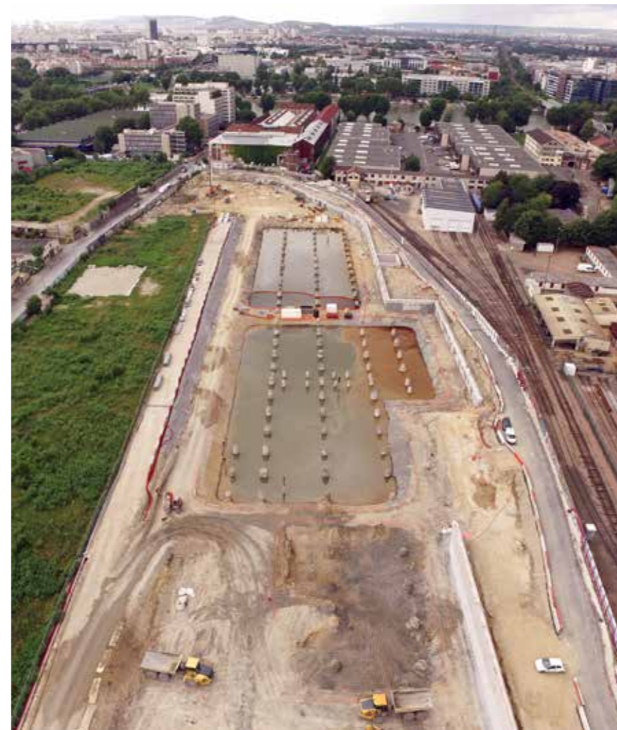
In Saint-Ouen (France), GRS Valtech cleaned up ground set to accommodate the maintenance and storage site for carriages from the Paris metro’s line 14.
